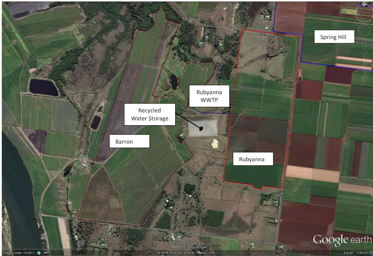
Figure 2-7: Recycled water storage location
