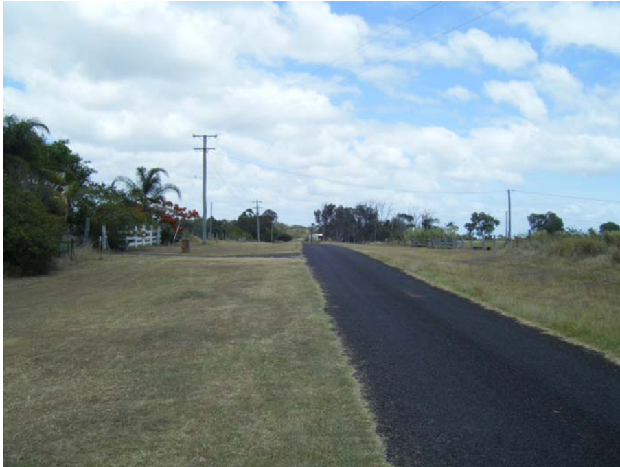
Photo 11 Outfall main location along Rubyanna Road
