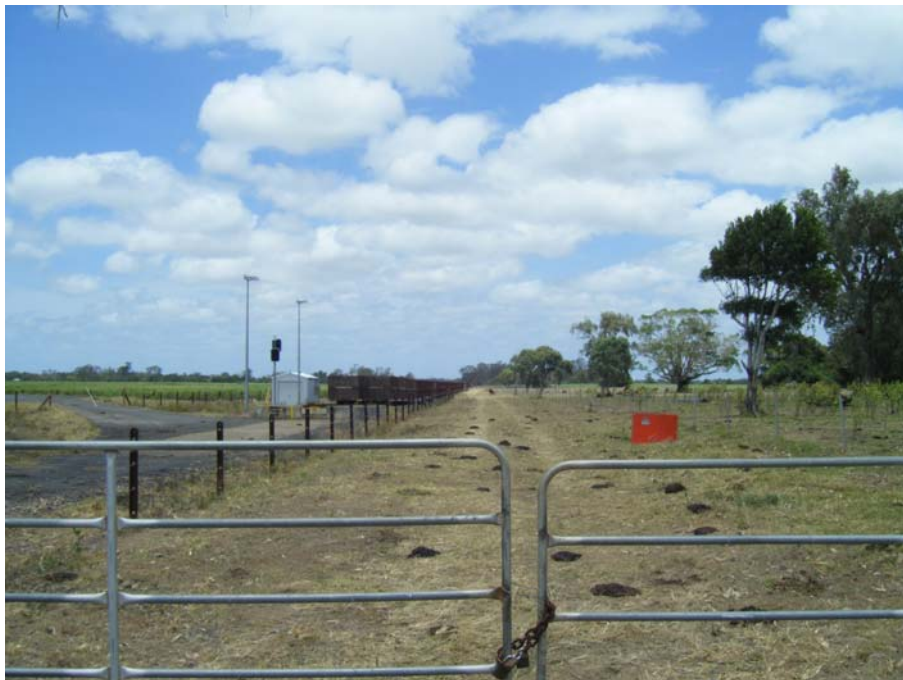
Photo 12 Outfall main location along Barrons Road Easement
