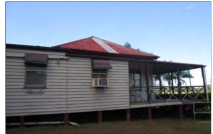
View to southern elevation.
