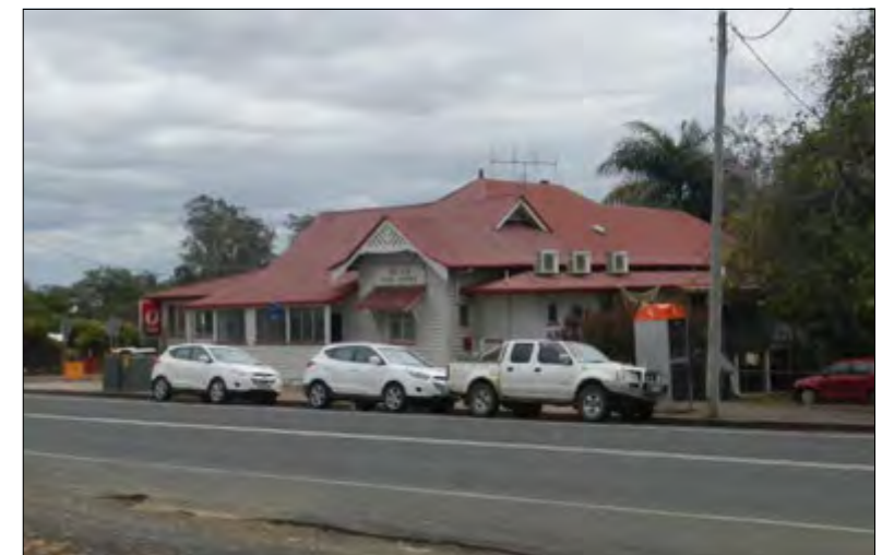
View to front and eastern elevation.
