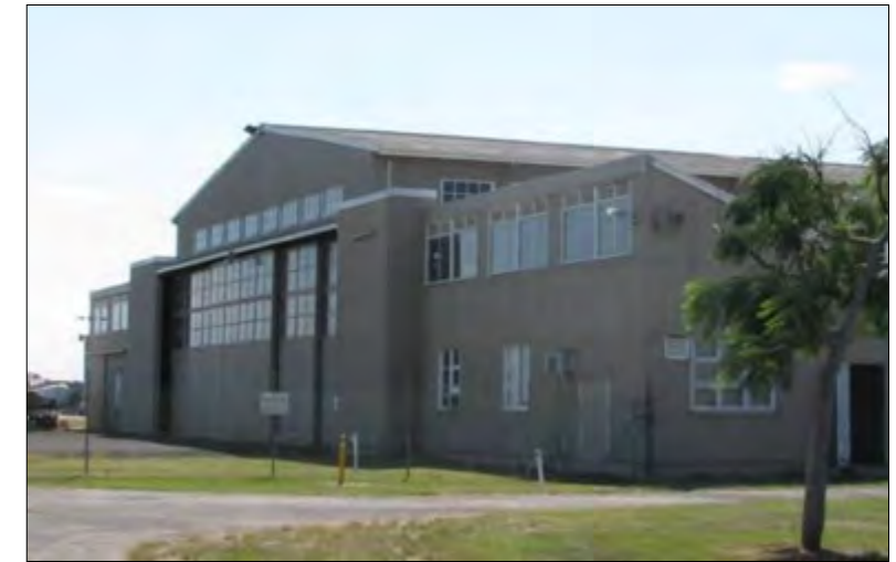
Hangar and workshop building.
