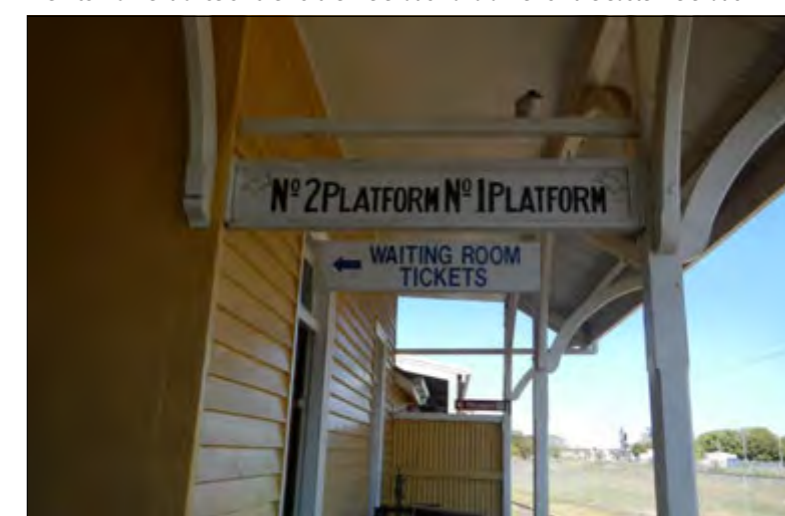
Close-up of platform awning.
