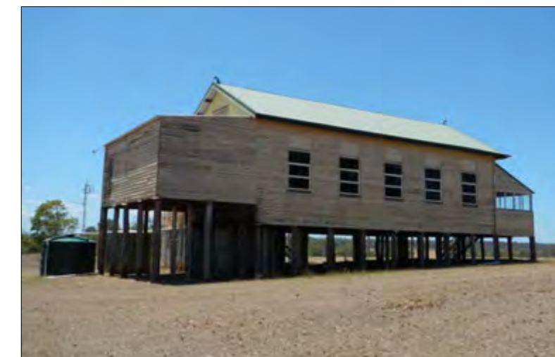
View to rear and southern elevation.
