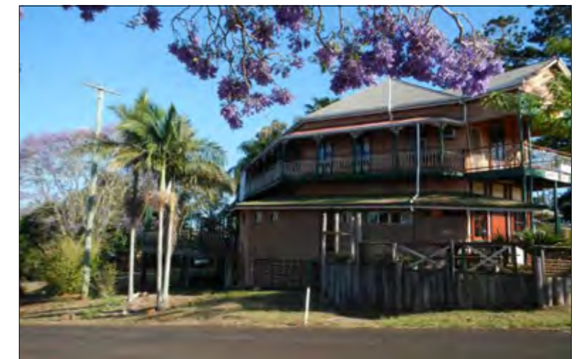
View to southern elevation.
