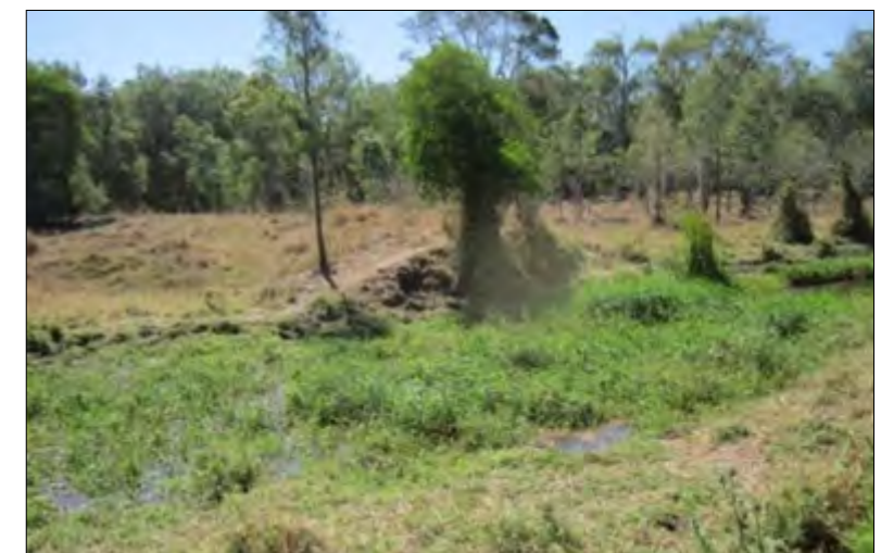
Evidence of former railway abutments in Cablehouse Creek.
