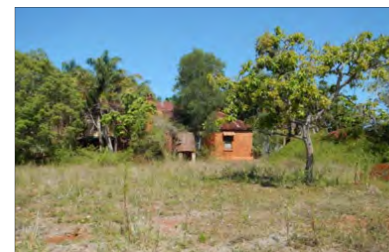
View to former dining room and kitchen.
