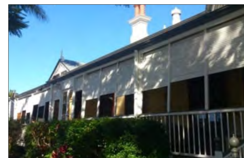
Eastern verandah detail.
