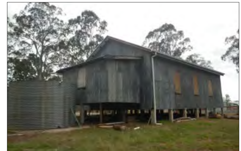
Rear and southern elevation.
