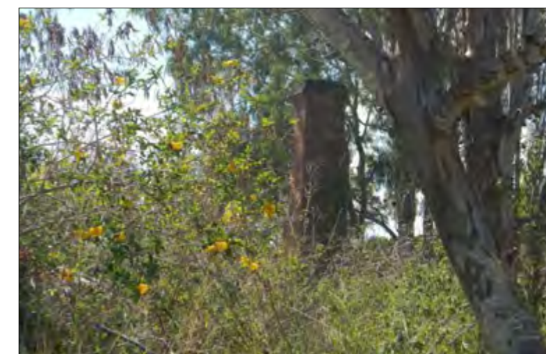
Brick chimney in the south-western section.
