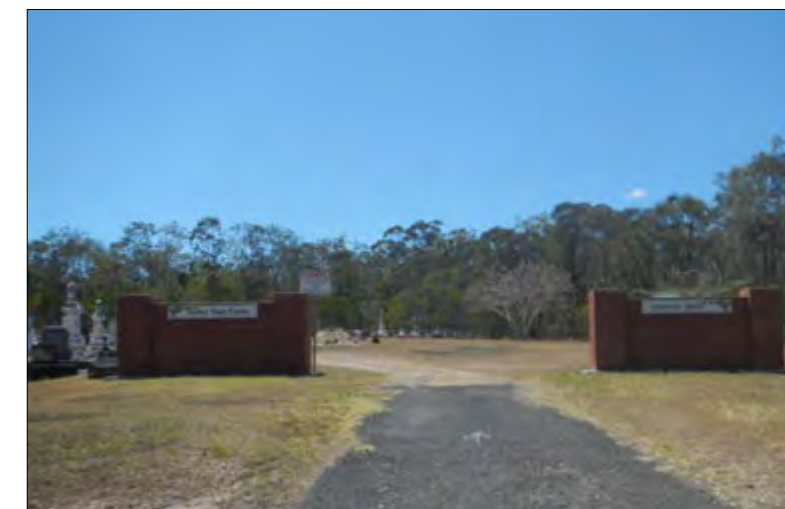
View to entrance.
