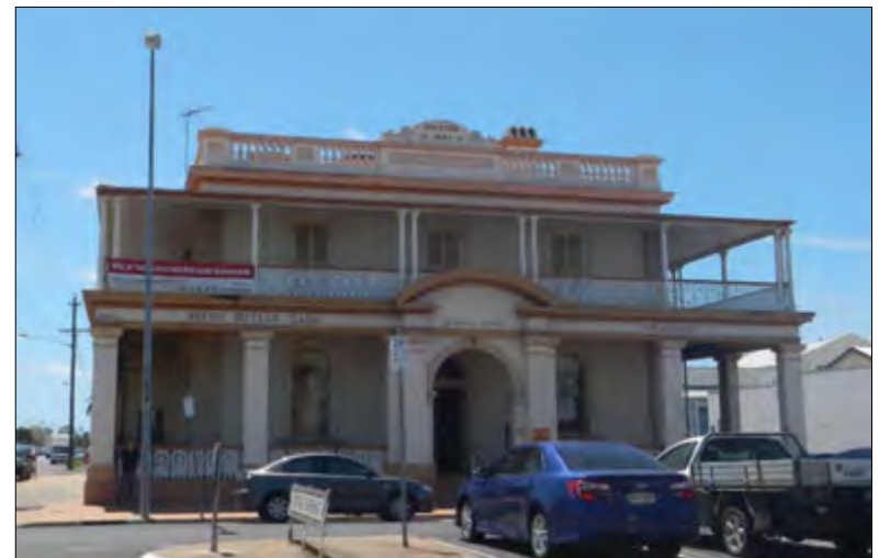
View to western elevation from Targo Street.
