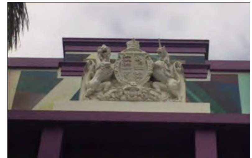
Cement Government Crest Quay Street frontage.
