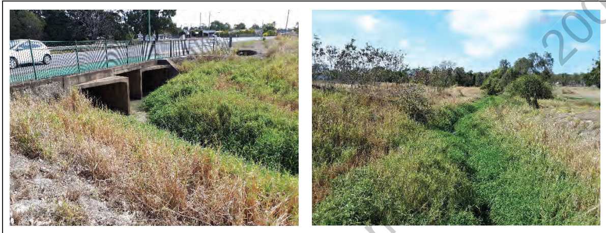
Figure 2 – Photos: Downstream of Fairymead Road Culverts (September, 2018)
