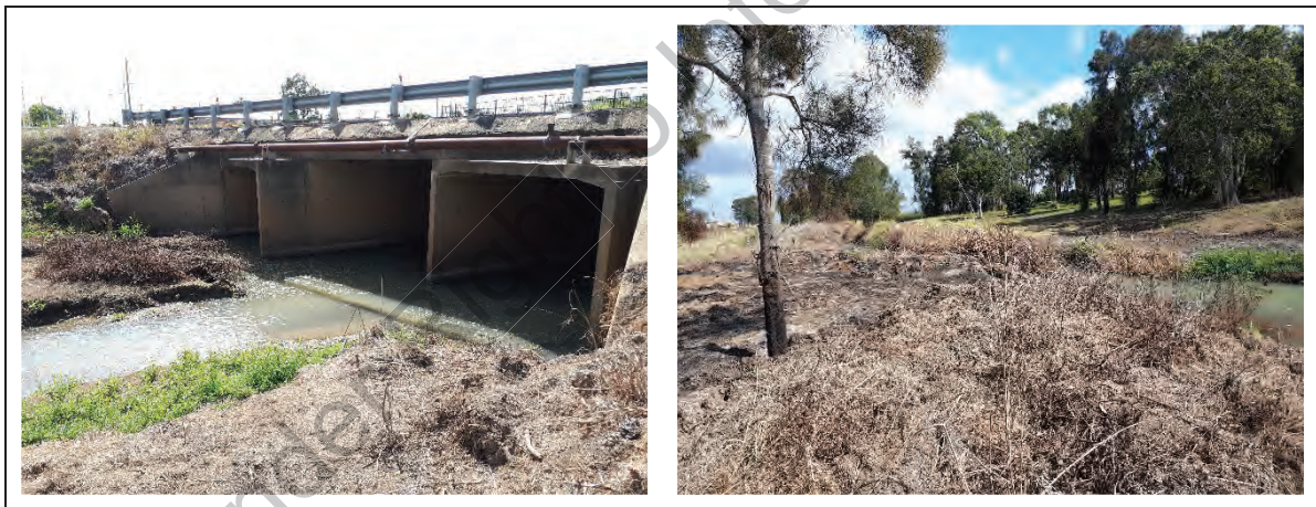
Figure 3 – Photos: Upstream of Fairymead Road Culverts (September, 2018)
