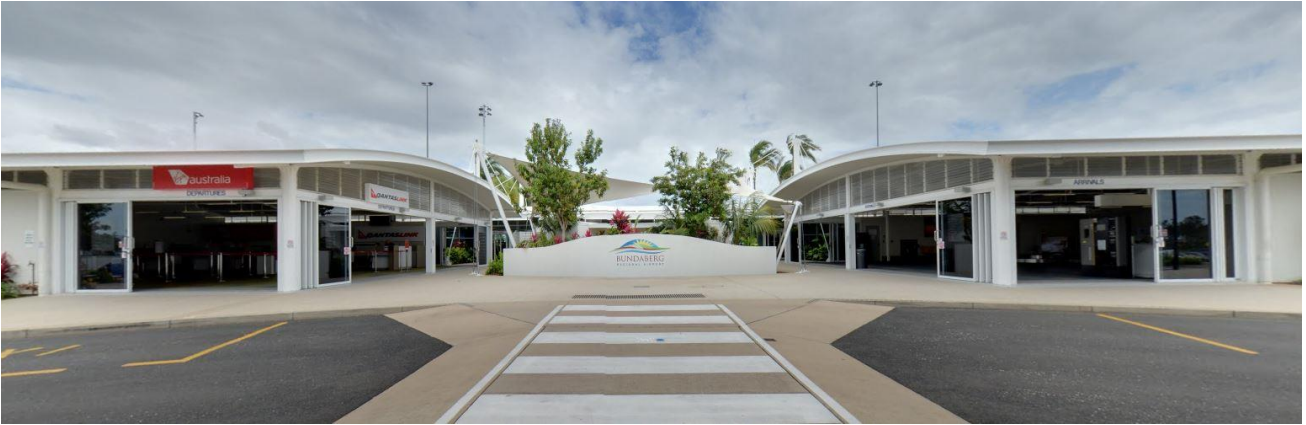
Image 2: Front of terminal (landside)
