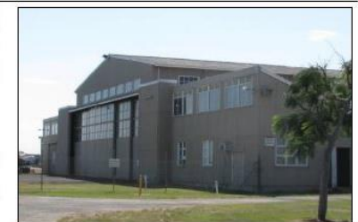
Hangar and workshop building.
