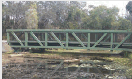
Baldwin Swamp Environmental Park Bridge
