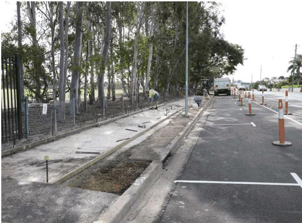
Pathway construction on Maryborough Street, Bundaberg.
