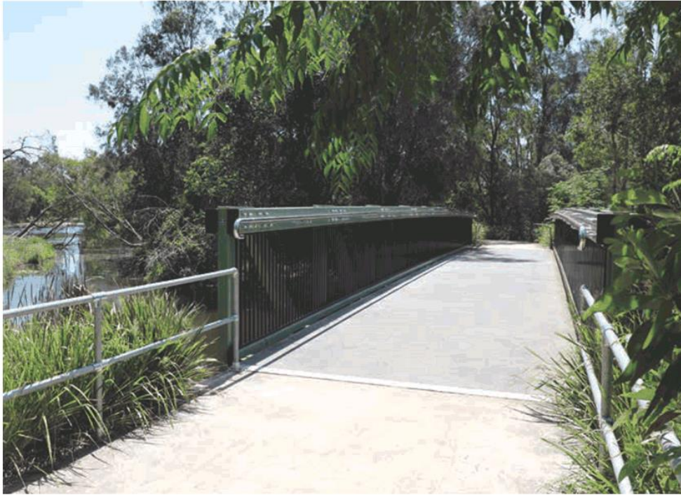
Bridge and pathway at Baldwin Swamp Environmental Park.
