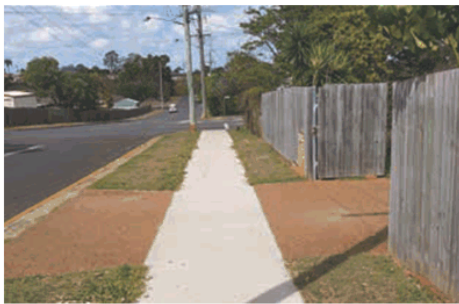
Photograph 1 – Pathway Constructed with Pathway Priority
