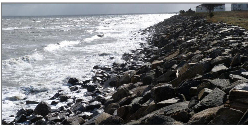
Figure 1 (above): Example of a similar rock seawall which would be built along the eastern side of Mariners Way.
