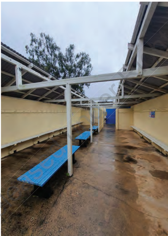
Figure 10: Interior Men's Dressing Shed (1956) (Queensland Government, 2022)
