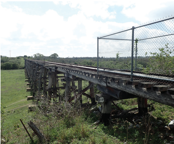
Splitters Creek Bridge
