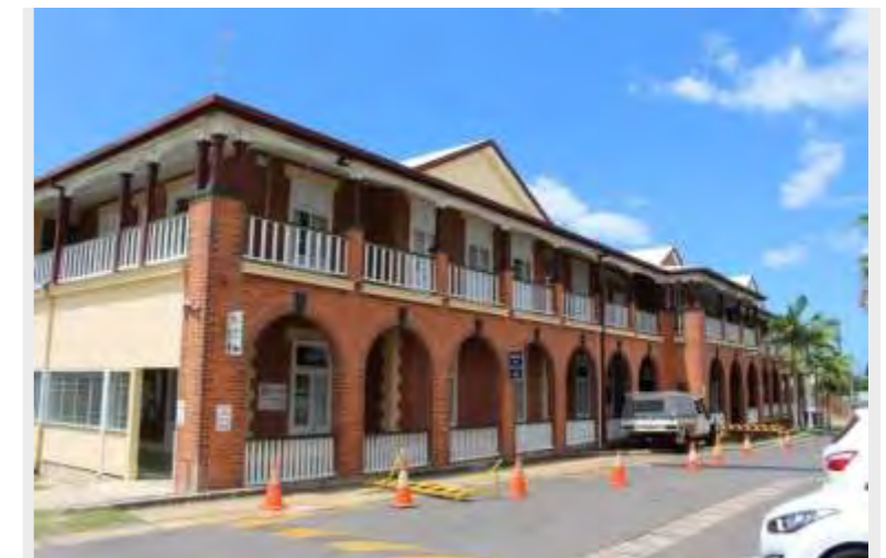
Southern elevation of Old Quarters.
