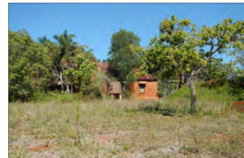
View to former dining room and kitchen.
