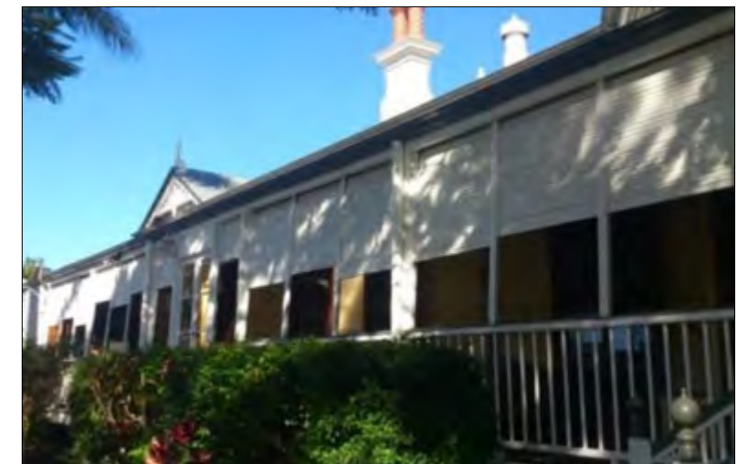
Eastern verandah detail.
