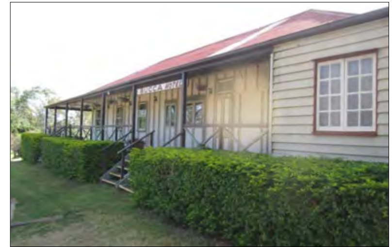
Entrance to Bucca Hotel, view to southwest.
