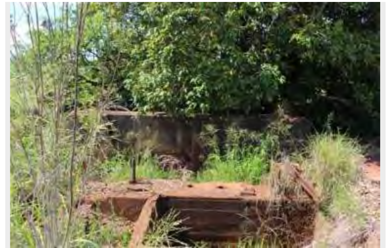
Footings of crushing plant.
