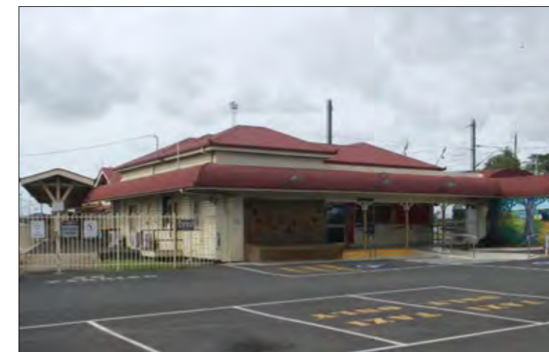
View to entrance from carpark.
