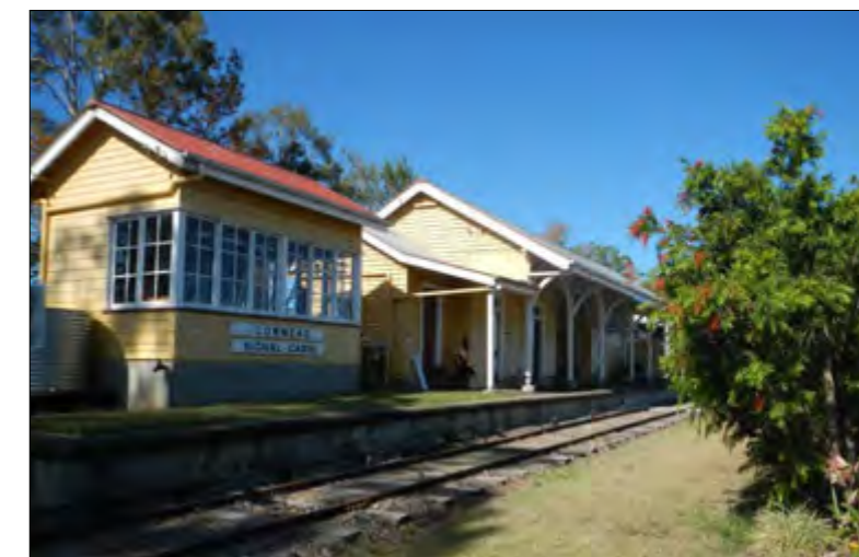
View to railway station and signal cabin from the south.
