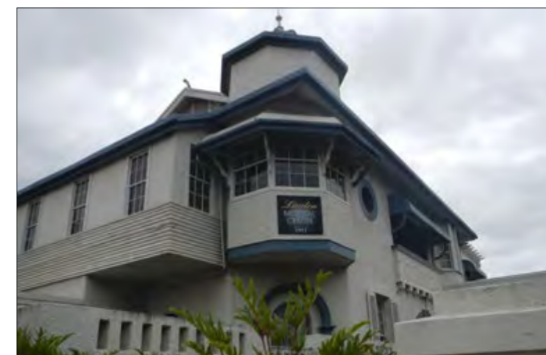
Close-up of turret element above original entrance on southeast corner.
