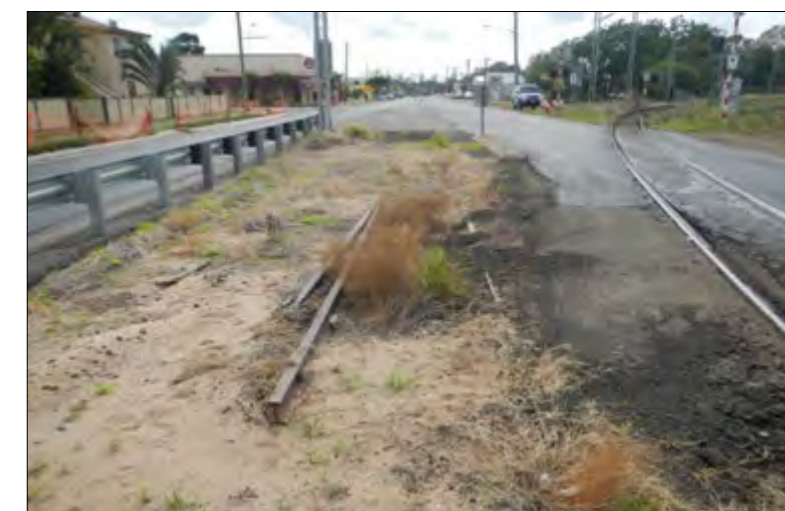
Turn-off section of the North Coast Railway Line, looking east.
