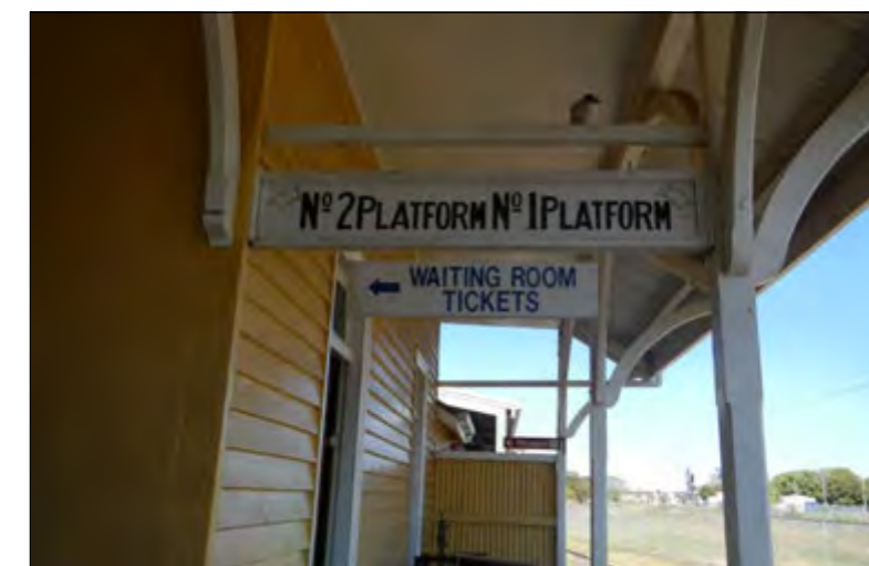
Close-up of platform awning.
