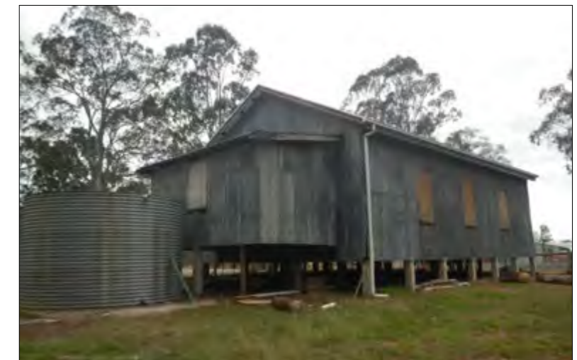
Rear and southern elevation.
