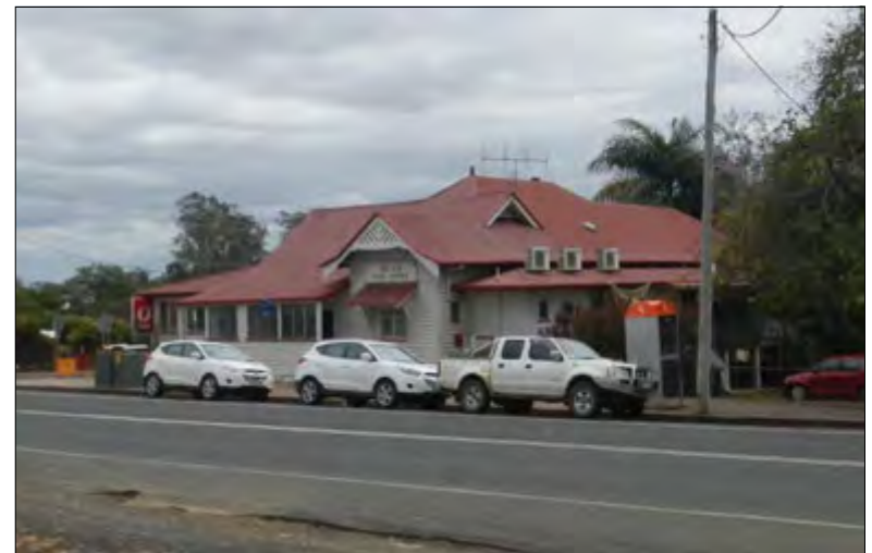
View to front and eastern elevation.
