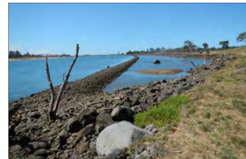
View to the wall from the south.
