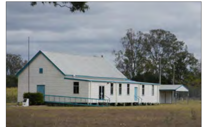
View to front and eastern elevation.
