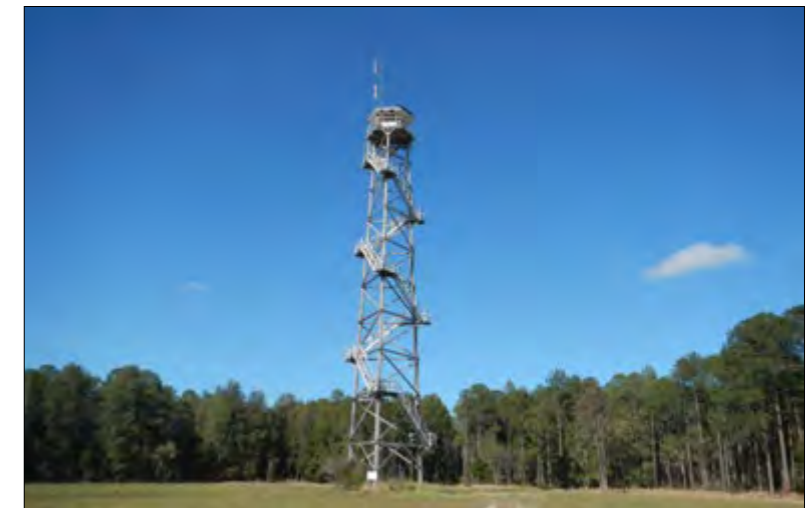
View of fire tower and setting.
