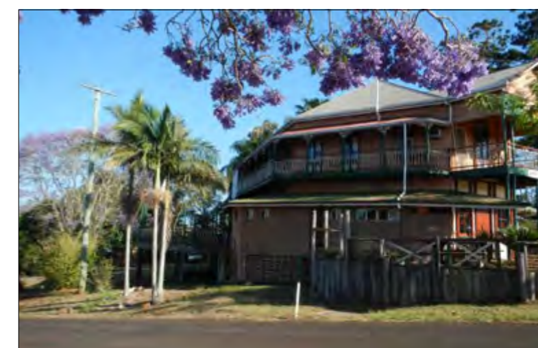
View to southern elevation.
