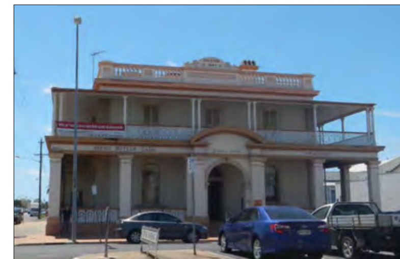
View to western elevation from Targo Street.
