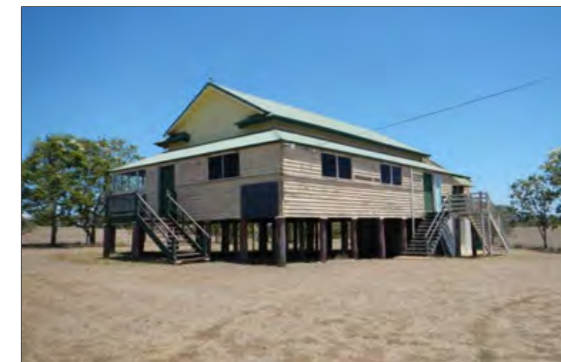
View to front and northern elevation.
