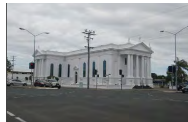
View to front and northern elevation from corner Woongarra and Barolin Streets.
