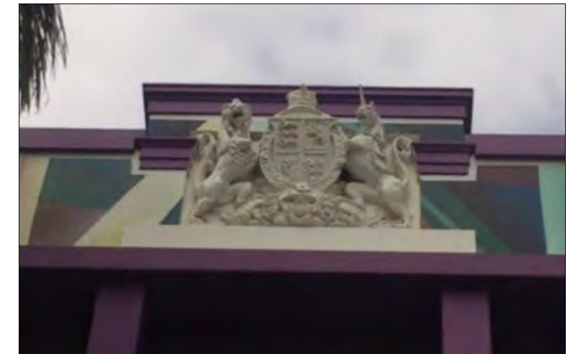
Cement Government Crest Quay Street frontage.
