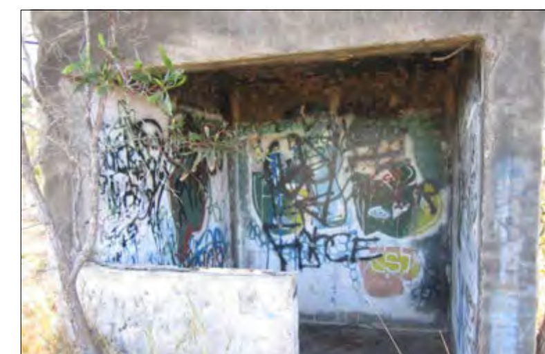
Close-up of door entrance and observation window.
