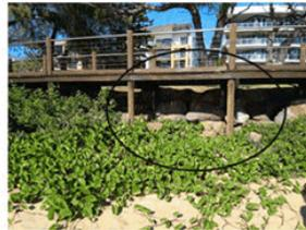
The area behind the boardwalk is variably eroded with small, localised scour pockets between rocks.
