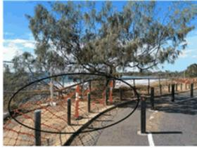
The shared path is undermined, and temporary safety fencing has been installed for safety reasons.
