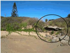
Scour hole behind the boat ramp abutment. Loosely placed rocks have been used to protect the eroded sections of the abutment.
