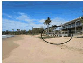
Existing revetment in front of the SLSC is providing a level of protection but erosion threat may increase with sea-level rise and increase in storm intensity.
