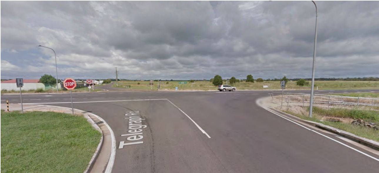
Figure 8: Western Approach to Telegraph Road – Bundaberg Ring Road Intersection (Source: Google Streetview, 2020)
