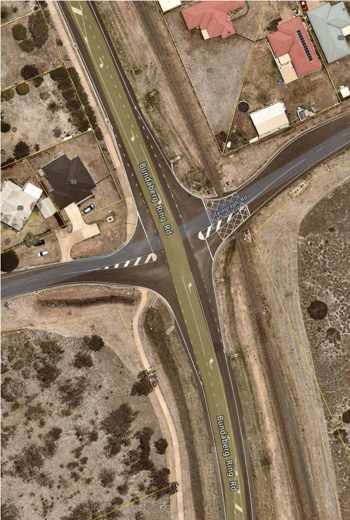
Figure 5: Telegraph Road – Bundaberg Ring Road Intersection (Source: Nearmap, 2020)
