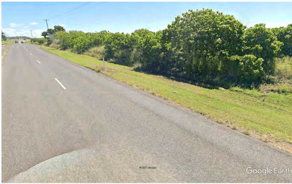
Photograph 1 – Existing table drain on Rifle Range Road (source: Google Earth)
