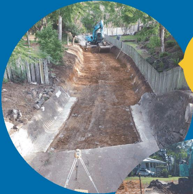
Maintenance on existing stormwater channel
