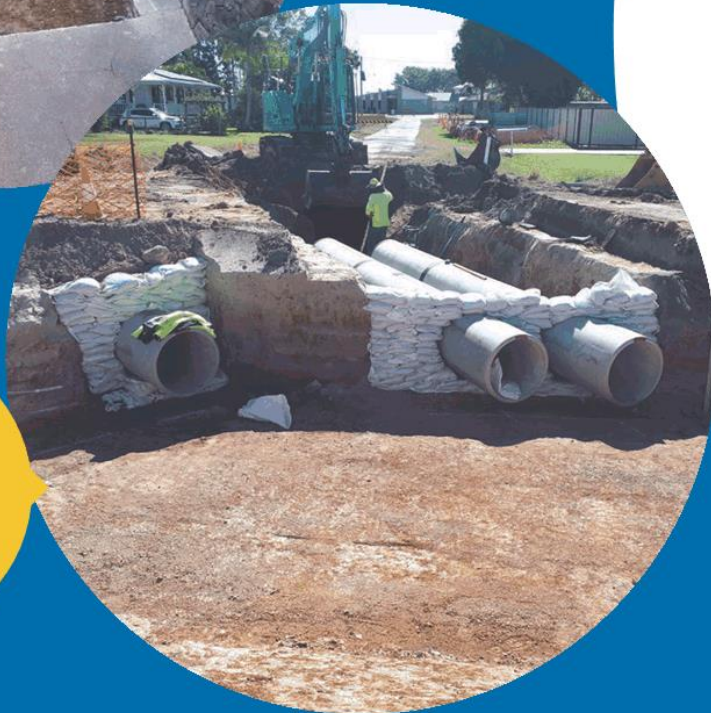
New stormwater pipe construction
