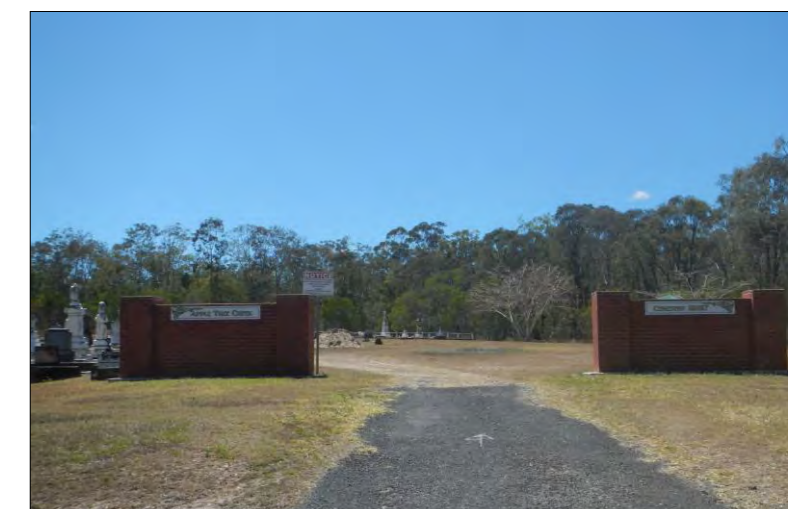
View to entrance.
