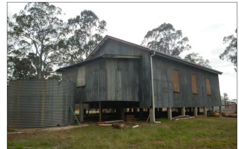
Rear and southern elevation.
