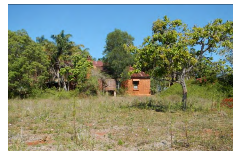
View to former dining room and kitchen.
