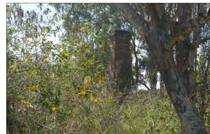
Brick chimney in the south-western section.
