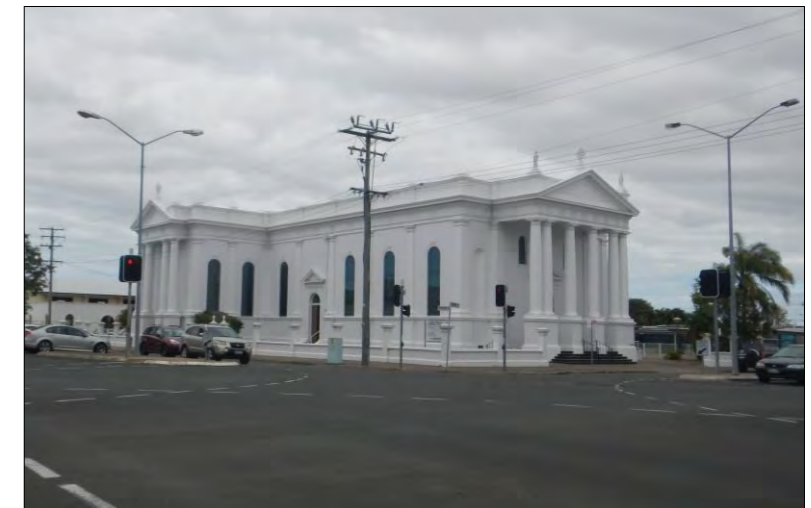
View to front and northern elevation from corner Woongarra and Barolin Streets.
