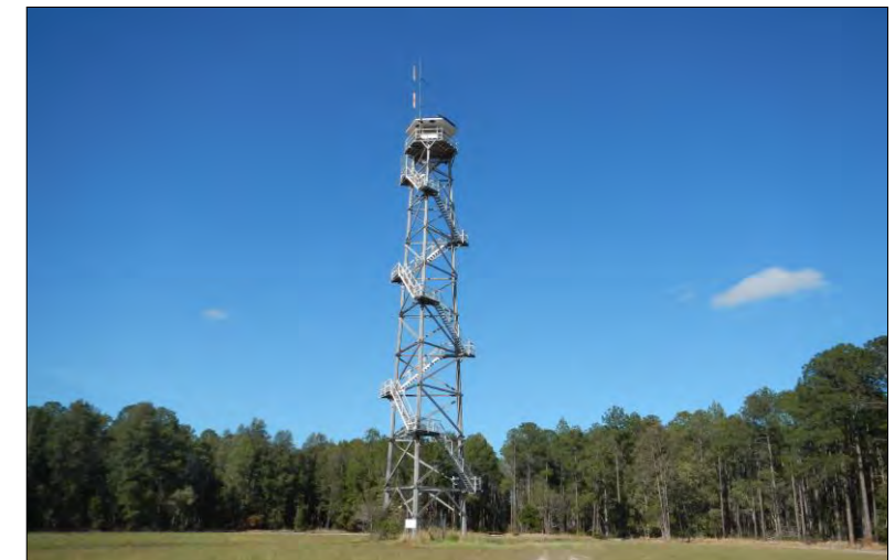
View of fire tower and setting.
