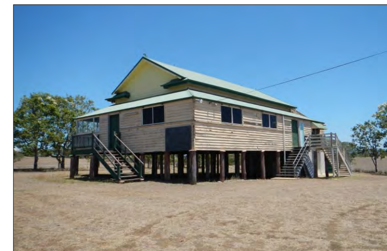
View to front and northern elevation.
