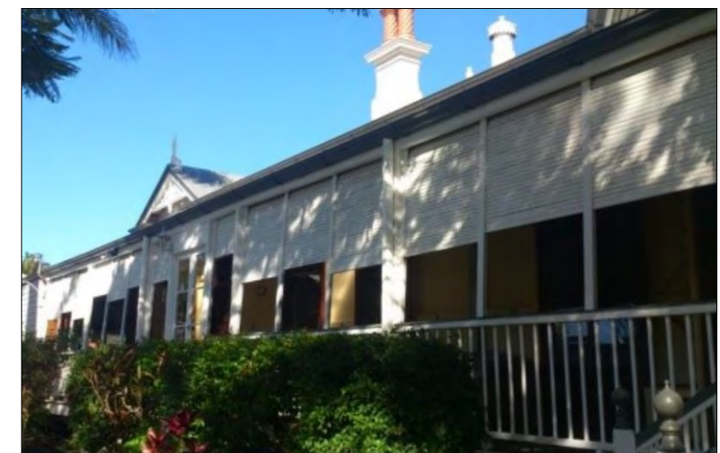
Eastern verandah detail.
