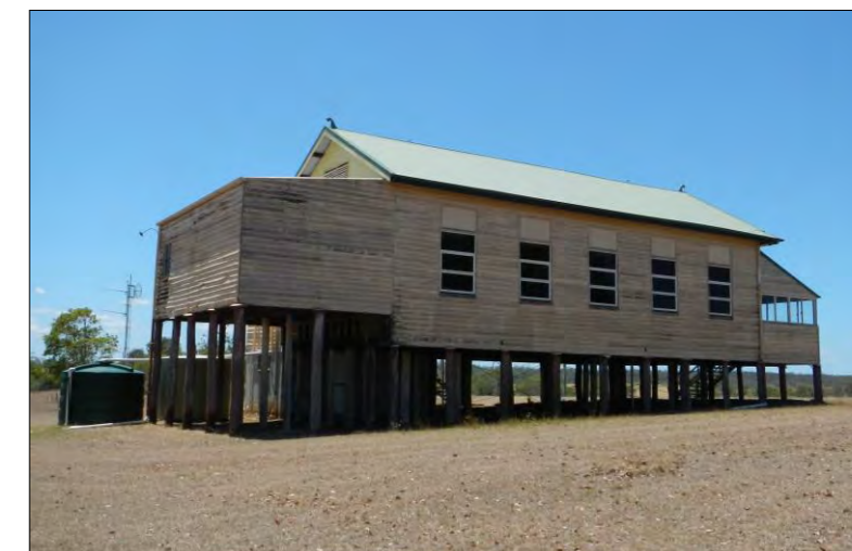
View to rear and southern elevation.
