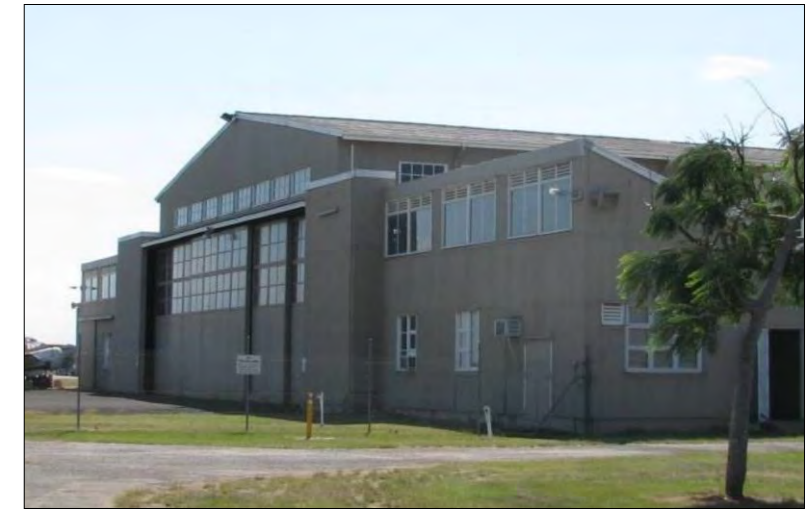
Hangar and workshop building.
