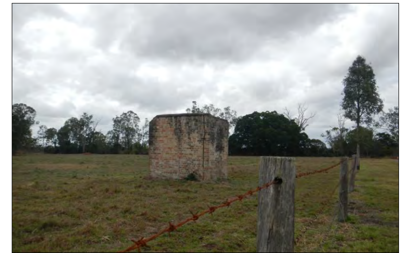
View to brick enclosure adjacent to Mill Road looking south.
