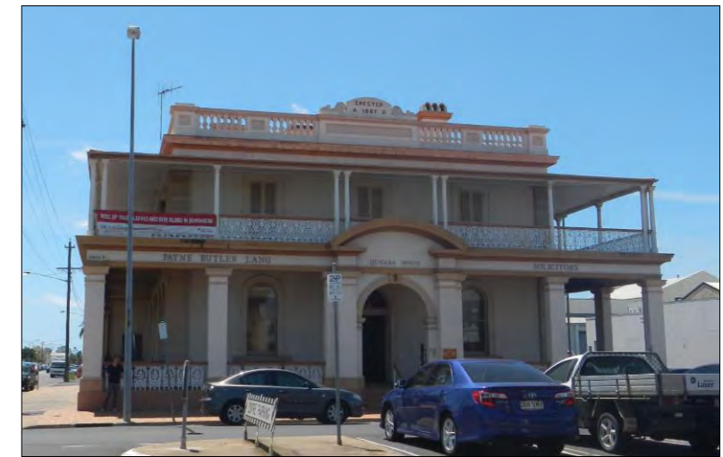
View to western elevation from Targo Street.
