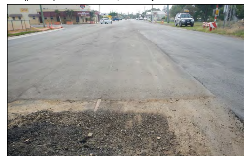
View of partially exposed railway tracks on Perry Street, looking east.
