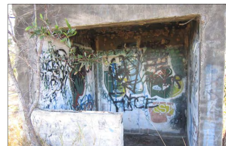
Close-up of door entrance and observation window.
