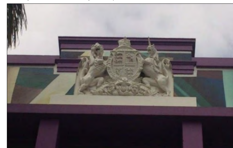
Cement Government Crest Quay Street frontage.
