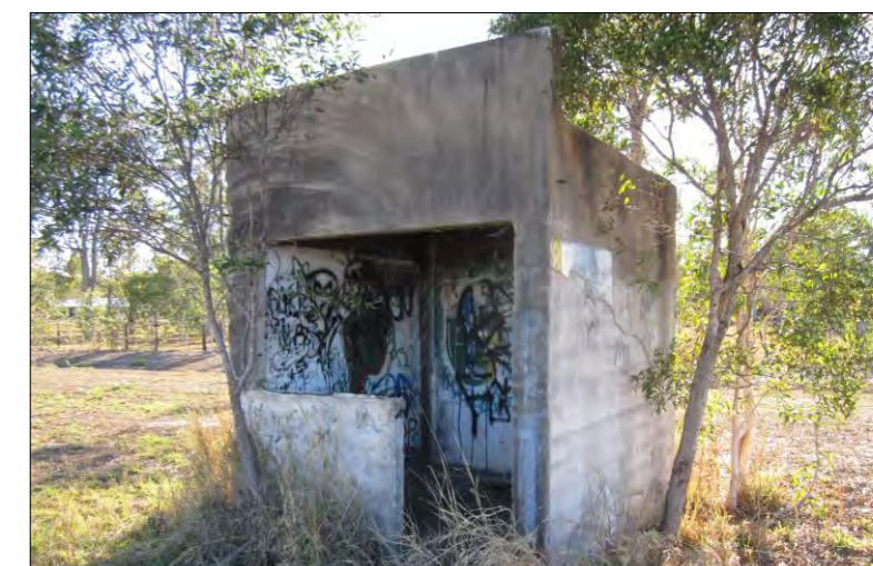
Door entrance and observation window, view to west.
