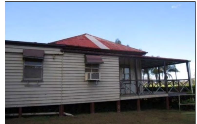
View to southern elevation.
