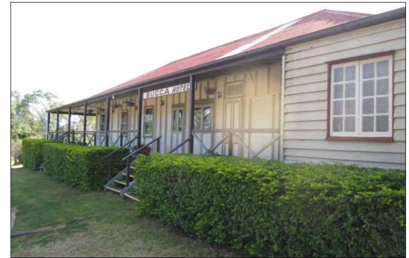
Entrance to Bucca Hotel, view to southwest.
