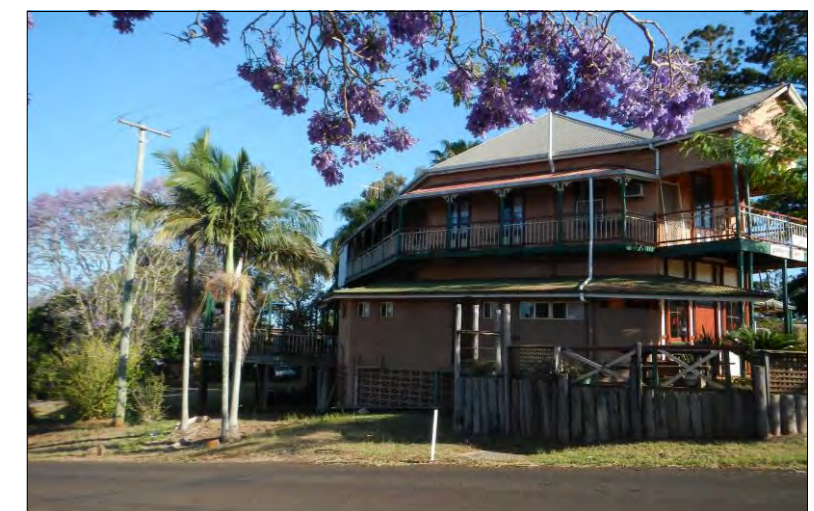
View to southern elevation.
