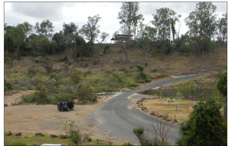
View to crossing from northern riverbank.
