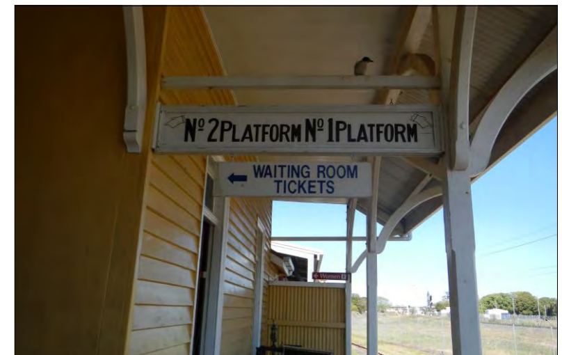
Close-up of platform awning.
