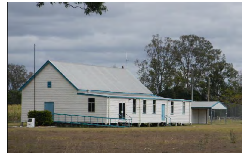
View to front and eastern elevation.
