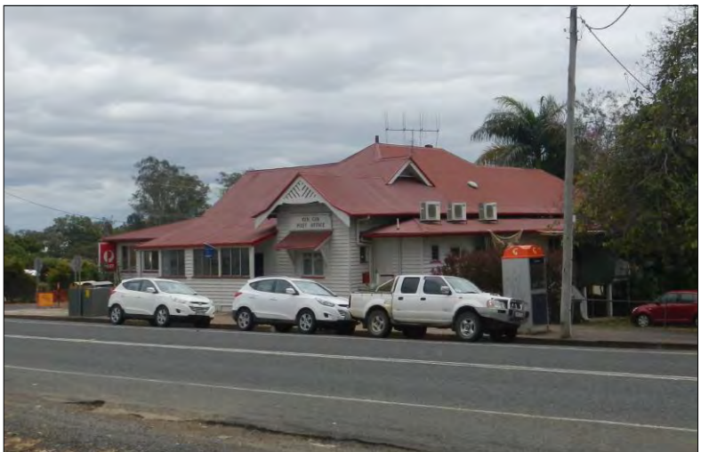
View to front and eastern elevation.
