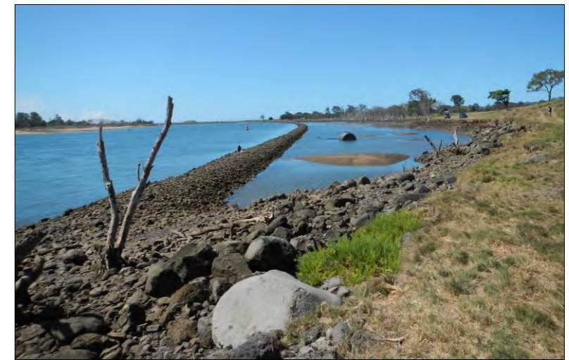
View to the wall from the south.
