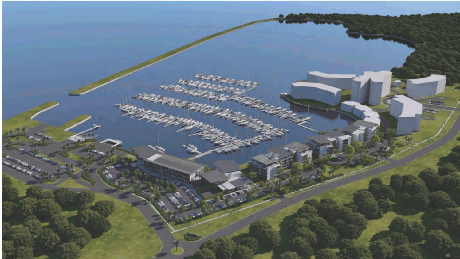
AERIAL VIEW OF PROJECT LOOKING SOUTH-EAST
