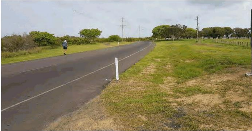
Figure 7-6: Access 2 looking north west
