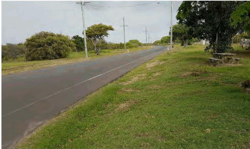
Figure 7-4: Access 1 looking north west
