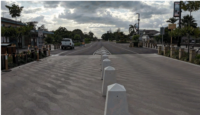
Figure 3-4: Zunker Street looking east
