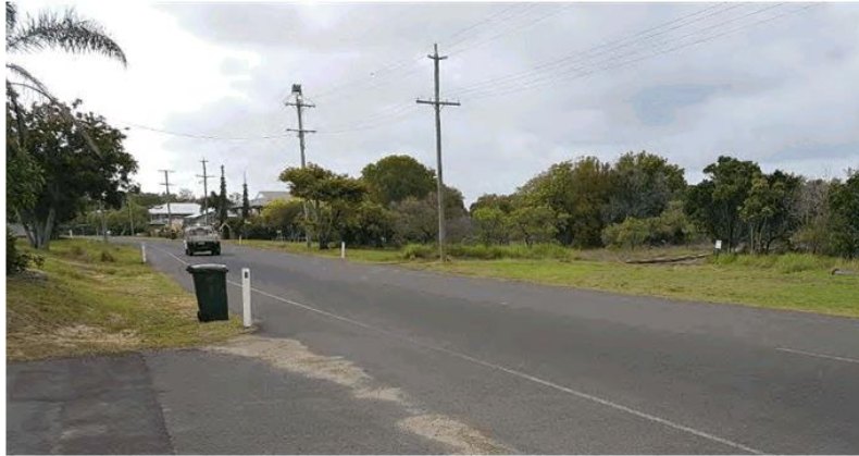
Figure 7-7: Access 2 looking south east
