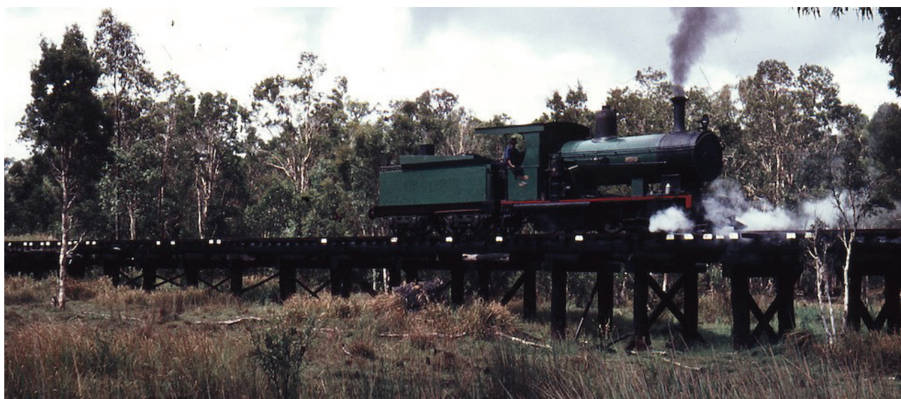
This bridge near Bingera Siding was typical of the 40 “flood openings” on the railway between Bundaberg and Gin Gin. Replacement of these missing structures will be a major cost component of the development of the proposed rail trail.
