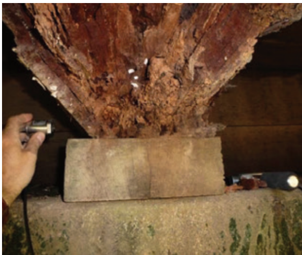
Figure 6-1: Photos showing global failure of a timber log girders. Both failures were caused by advanced decay in the ends of the girders and transverse shear failures. The primary cause of this decay was due to vertical fasteners. These failures were found in elements with SWT values in the 3k \mu s (photos a. above) to 6k \mu s range (photos b. below). Typically similar bending extreme tensile fibre failures in log girders occur in zones of decay where there are over 2k \mu s SWT values. Similarly if vast portions of the log girder have SWT values over 3k \mu s the failures may occur.
